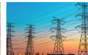
Electrical Temperature Measurement
